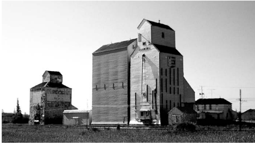
Figure 1: Fleming, Saskatchewan. This photograph displays three different shapes used in the construction of country elevators. On the left is the earliest, a square elevator with a gable-roofed cupola, Pool B No. 1164. The other two United Grain Growers elevators, sharing the same railway siding, are taller in form with gable roofs. The machinery for elevating the grain is housed in the cupolas. This photograph was taken in 1996; now only the oldest elevator, a heritage building, remains standing.
